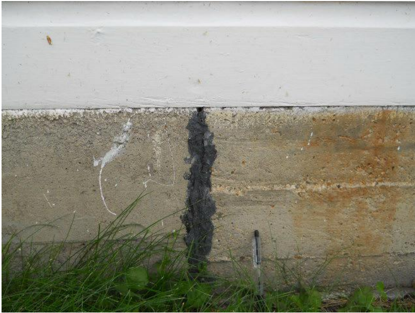
8/25/2011 10:46:45 AM View South of North Foundation Wall. Repaired Crack Visible (Crack 2) 505 Platt Avenue South, Red Lodge, MT 2011-0084.JPG
