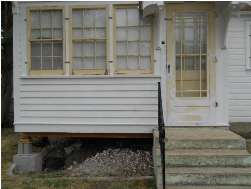
8/25/2011 10:41:38 AM View West of Front Porch (East Side of House) 505 Platt Avenue South, Red Lodge, MT 2011-0082.JPG
