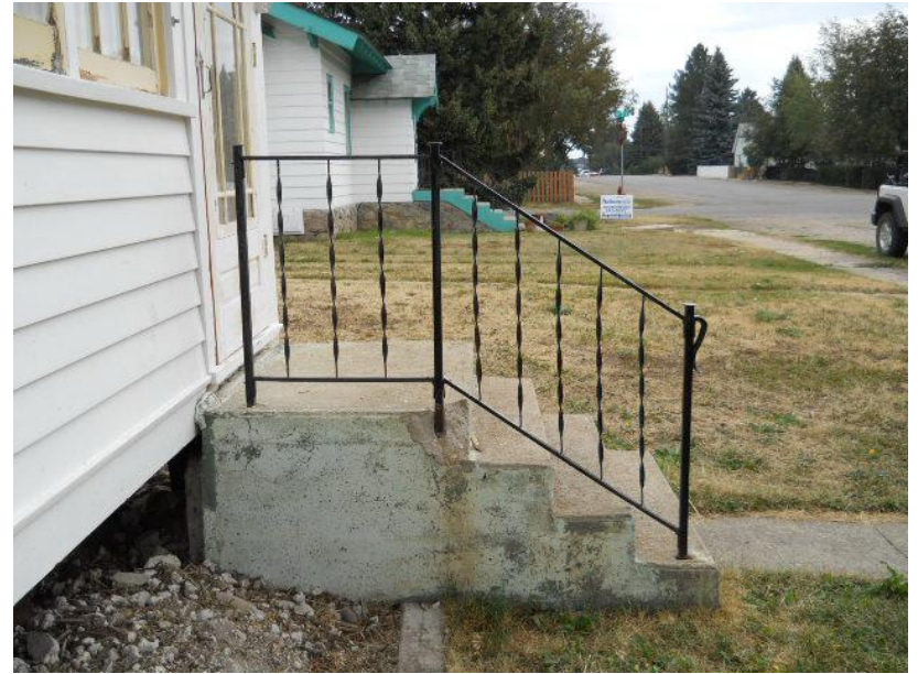
8/25/2011 9:55:20 AM View North of Front Porch of House 505 Platt Avenue South, Red Lodge, MT 2011-0073.JPG
