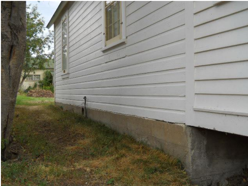
8/25/2011 9:56:08 AM View Northwest of South Side of House 505 Platt Avenue South, Red Lodge, MT 2011-0074.JPG
