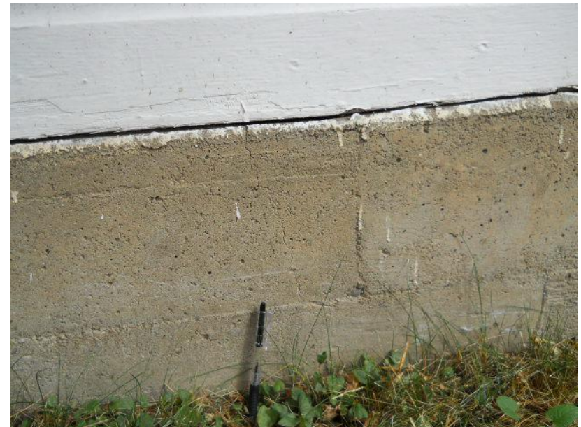
8/25/2011 10:46:01 AM View North of South Foundation Wall. Hairline Crack Visible (Crack 1) 505 Platt Avenue South, Red Lodge, MT 2011-0083.JPG
