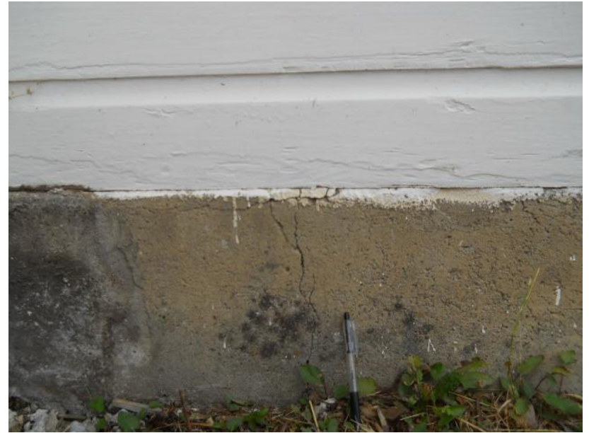
8/25/2011 10:47:07 AM View West of East Foundation Wall. Hairline Crack Visible (Crack 3) 505 Platt Avenue South, Red Lodge, MT 2011-0085.JPG
