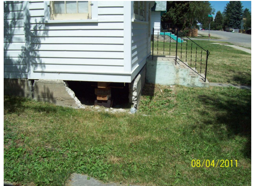
View North of the Porch Foundation Partially Removed 505 Platt Avenue South, Red Lodge, MT 100_2694.JPG
