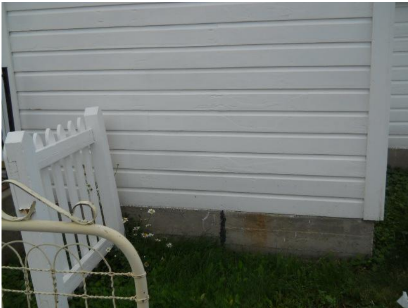
8/25/2011 10:39:00 AM View South of North Side of House. Note Patched Crack 505 Platt Avenue South, Red Lodge, MT 2011-0078.JPG
