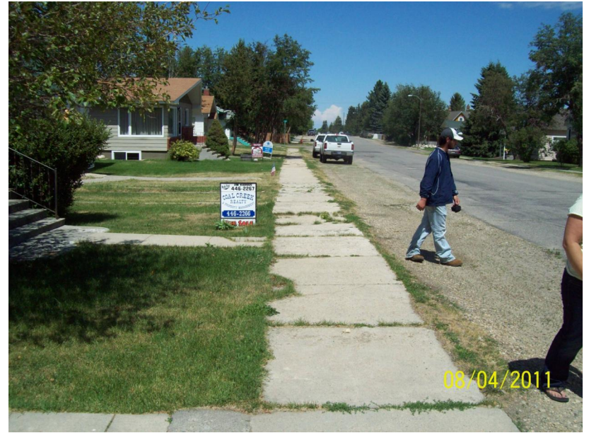
View North from South End of Block. View of Platt Avenue South and Sidewalk Platt Avenue South, Red Lodge, MT 100_2700.JPG
